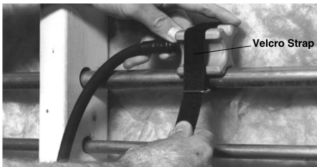
Figure 5 – Applying Freeze Head with Velcro Strap
